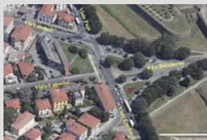
Present condition (aerial view)
