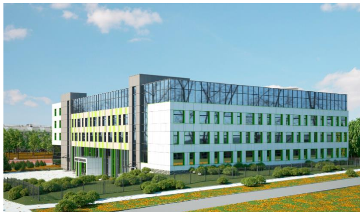
Main façade view with continuous glazing and the increased height of the first floor
