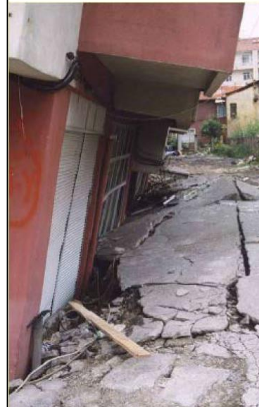
Izmit (Turkey), August 17, 1999 M7.4 earthquake
