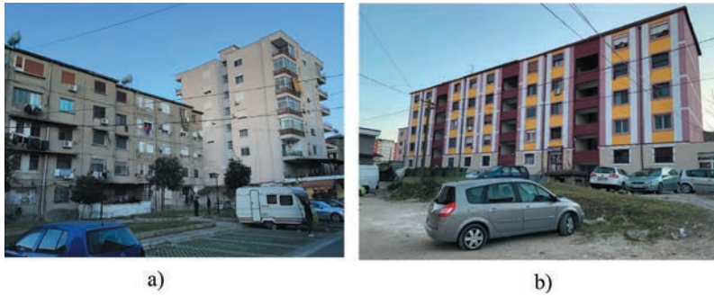
Figure 3. Typical LPE buildings in Albania: a) a typical 5-story LPE building and an adjacent 8-storey modern RC building, Durrës and b) a well-maintained and renovated LPE building, Vorë (photo: M. Baballëku).
