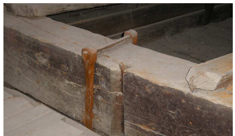
Connection of the truss tie - Jupiter dart
