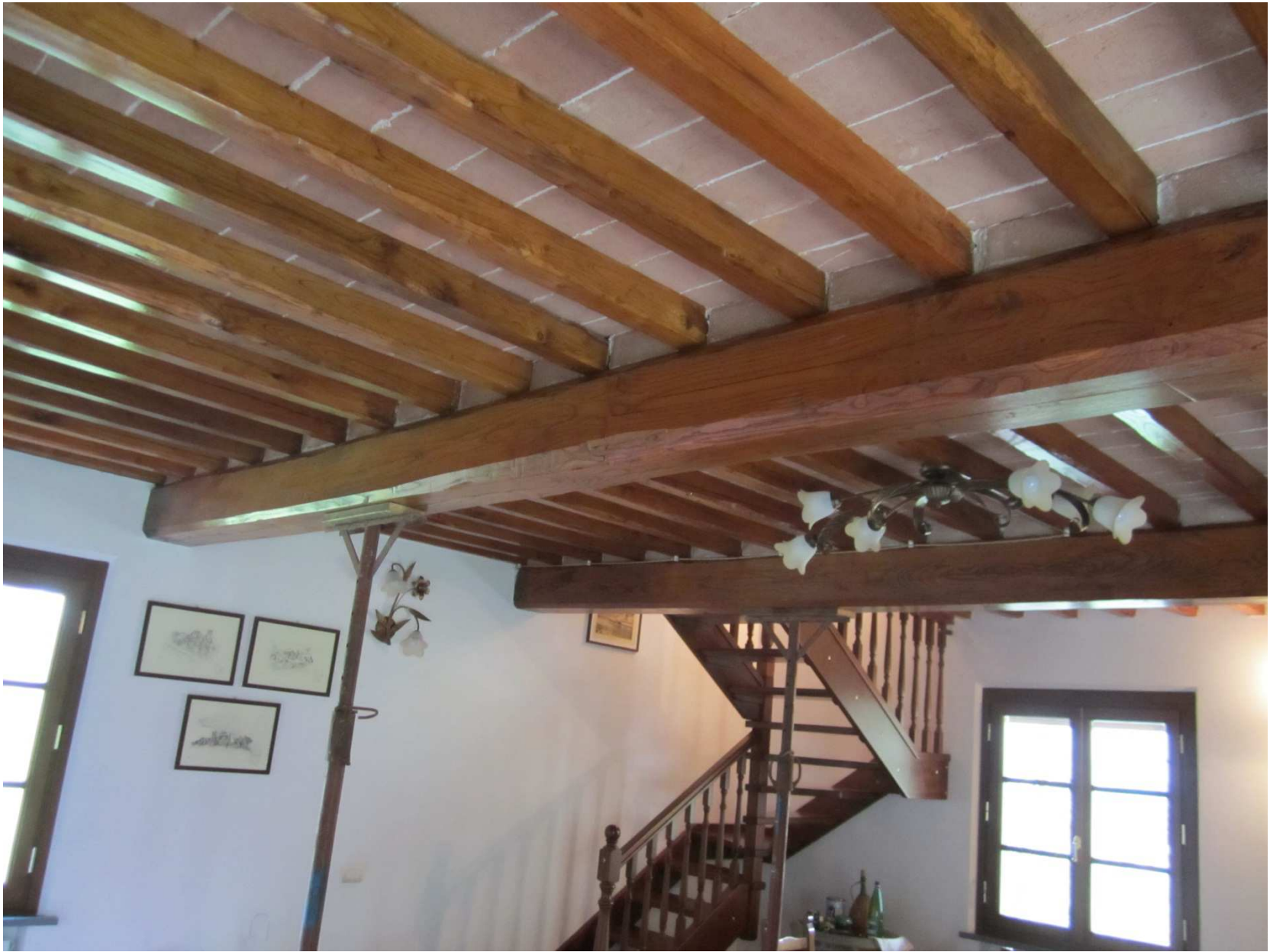
Beams supported with pack props
