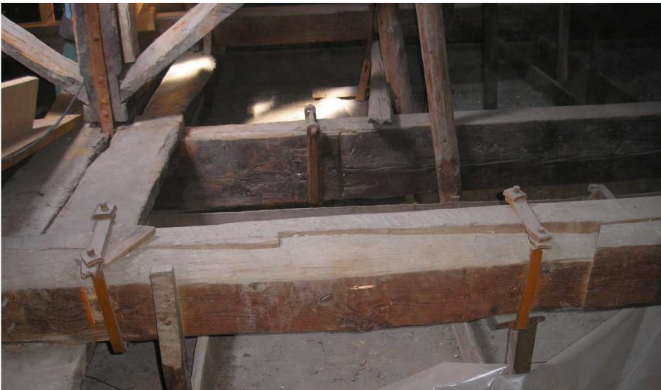
Connection of the truss tie - Jupiter dart
