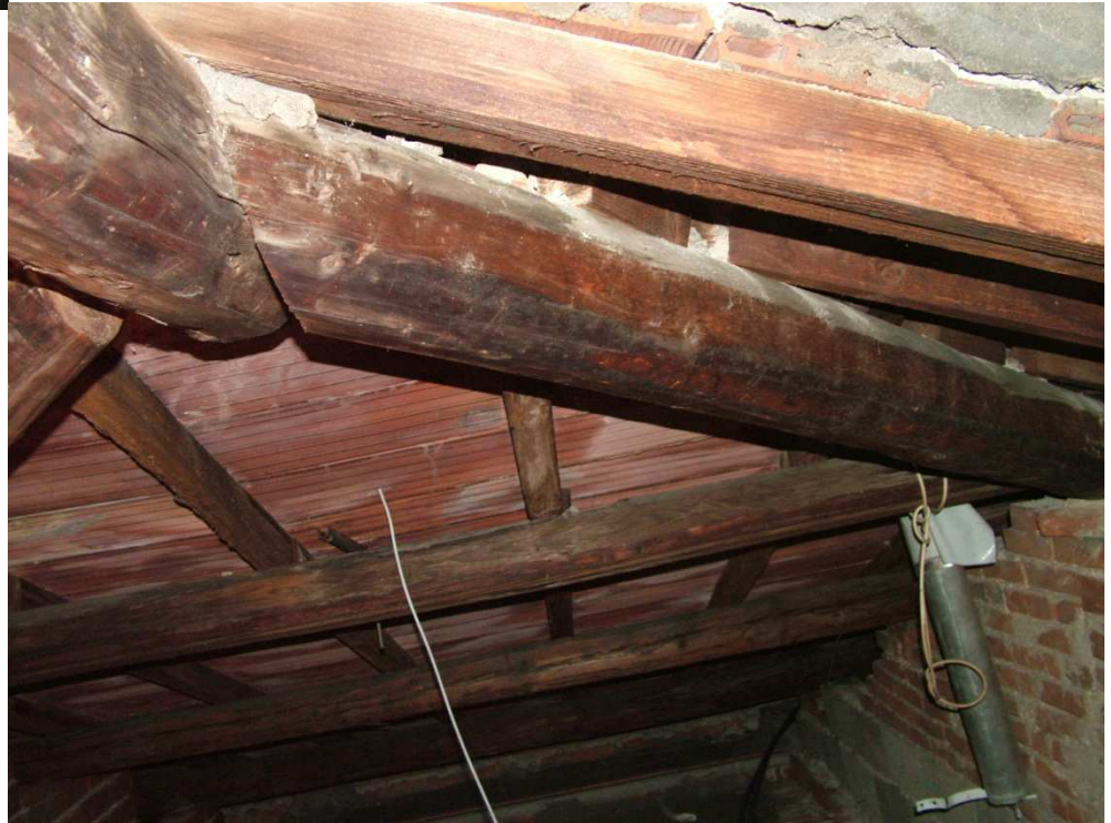
Cracked beam
