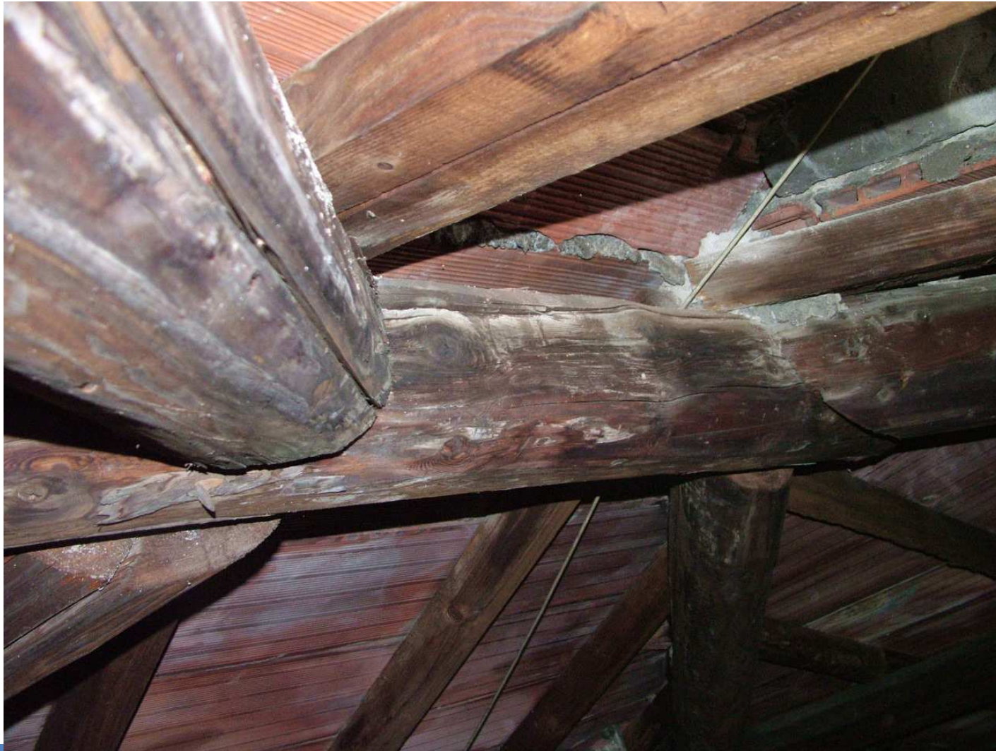
Cracked beam
