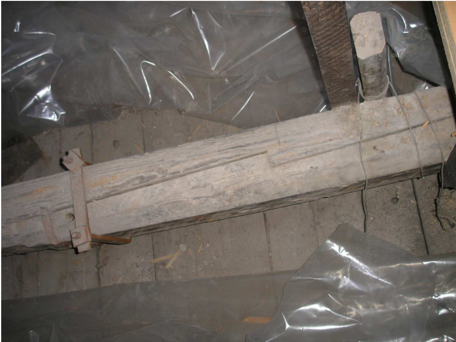
Connection of the truss tie - Jupiter dart
