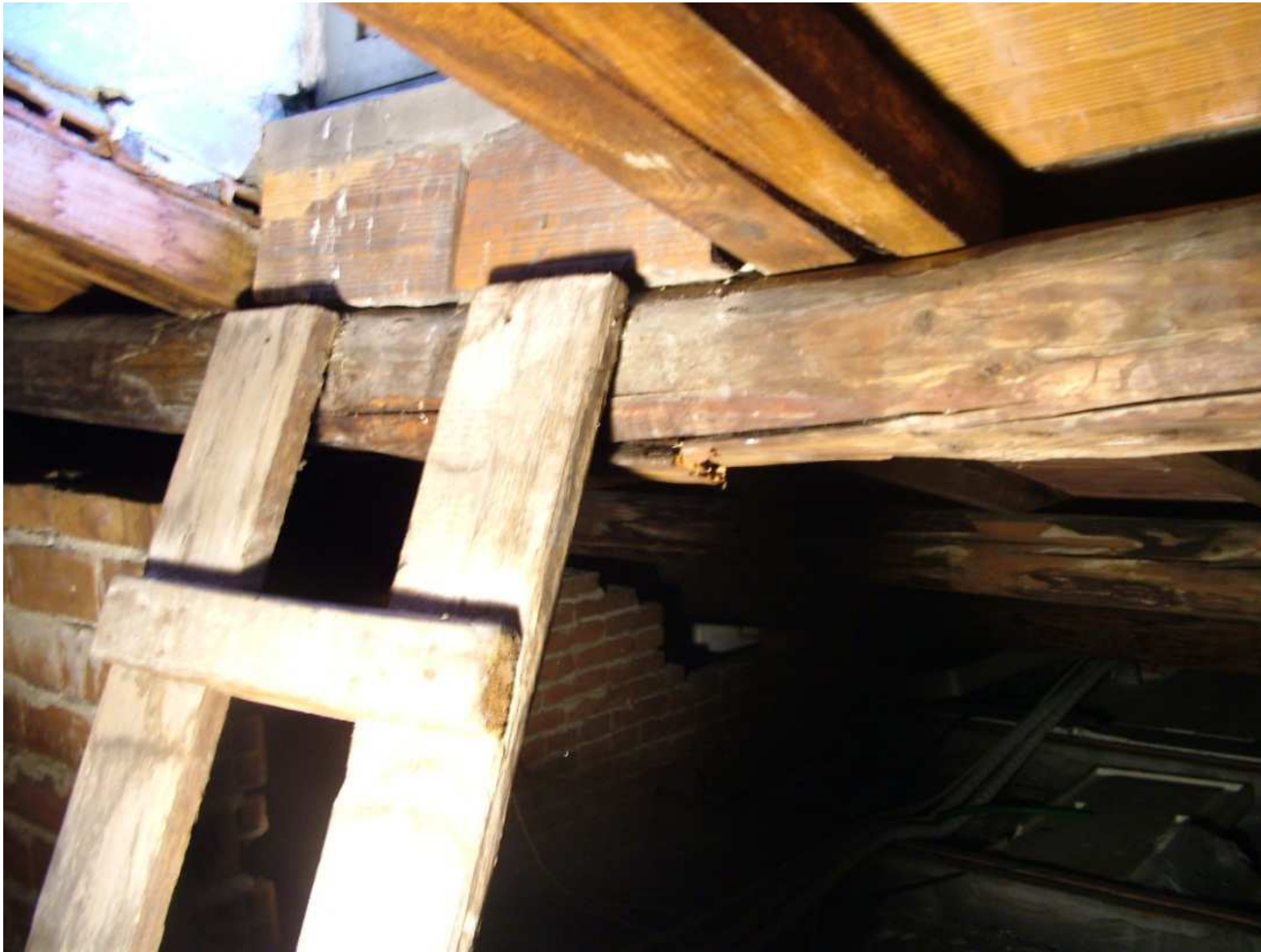
Cracked beam
