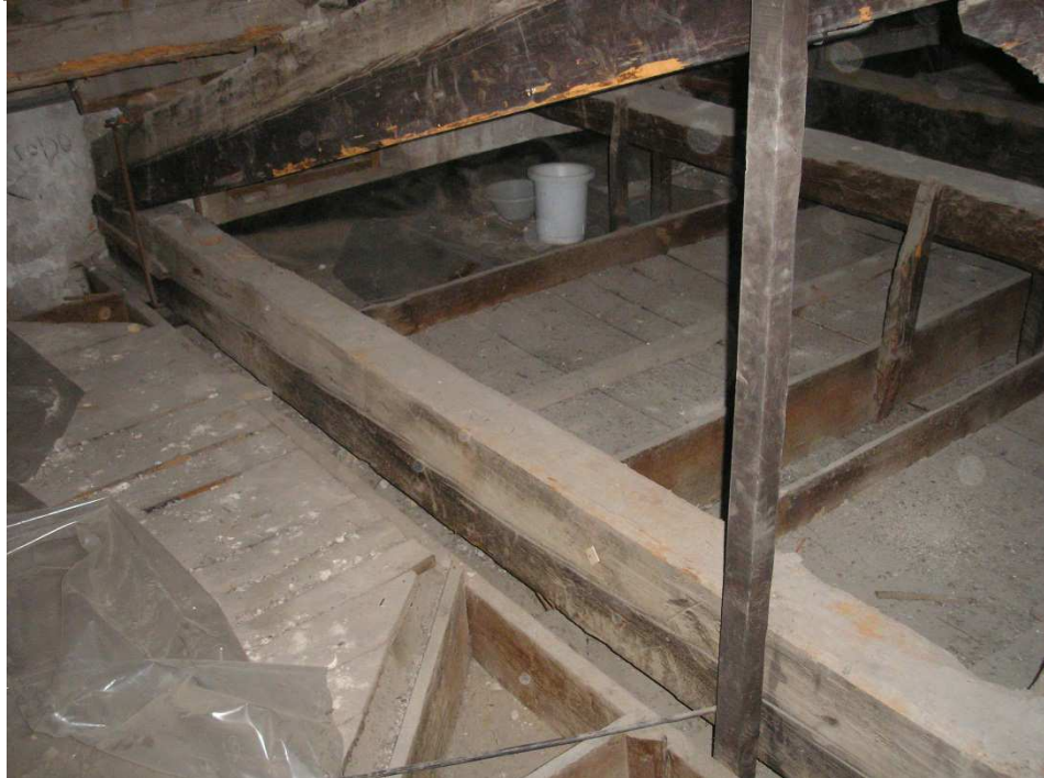
Suspension of the cieling
