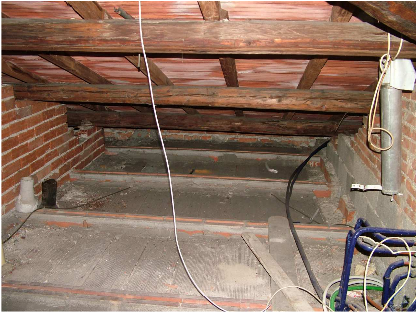
Cracked beam
