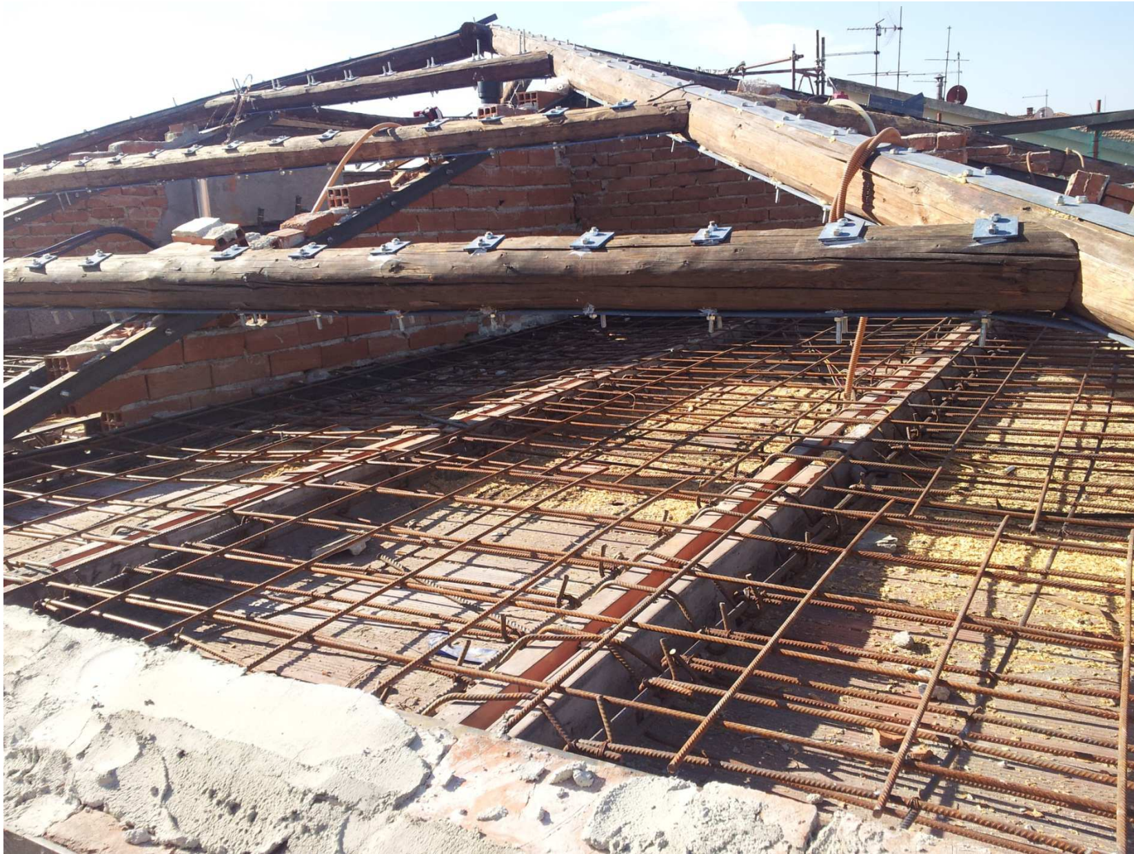
Strengthening of the roof during the works
