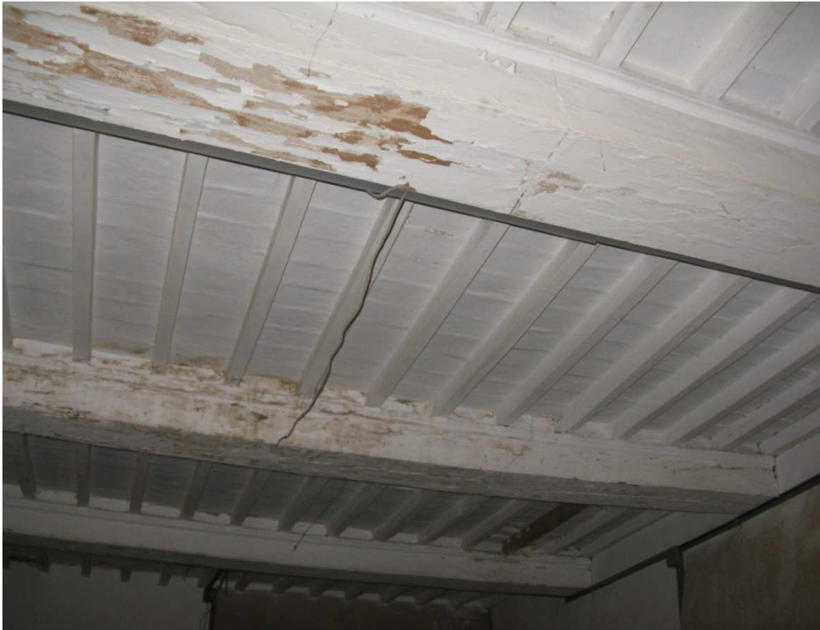
General view of the floor
