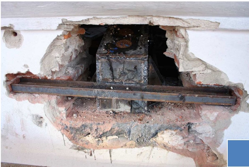
Repair of a damaged head
