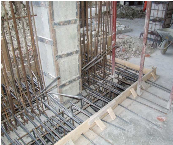
Execution of the shear walls
