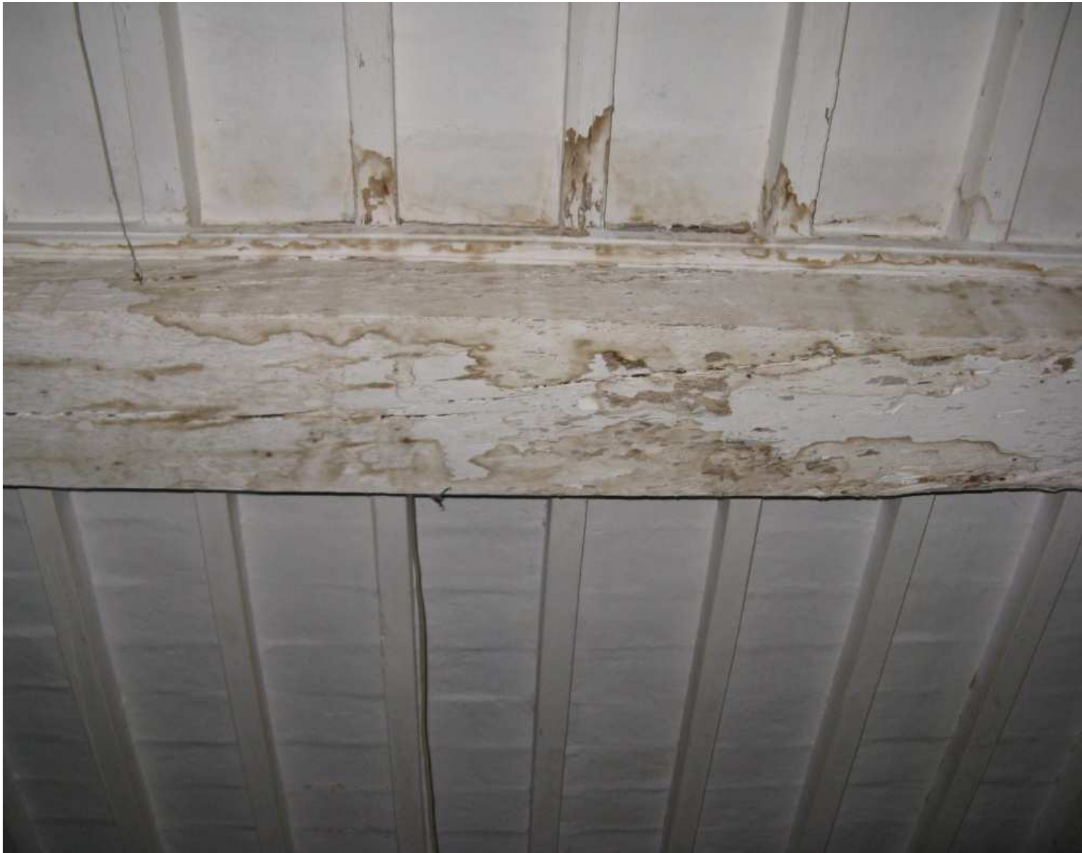
Crack pattern in a beam
