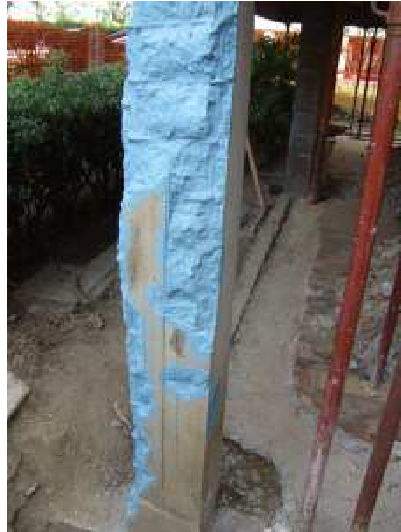
rust removal and passivation of the reinforcing bars
