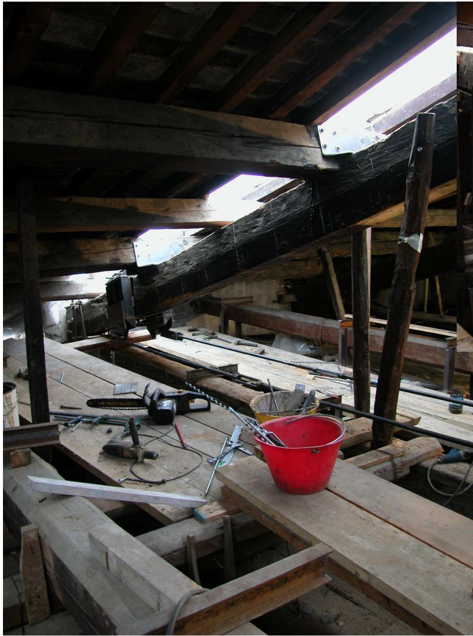
Repair of the truss and temporary chain
