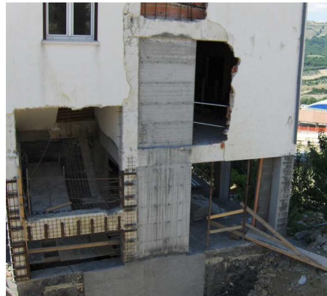
Execution of the shear walls
