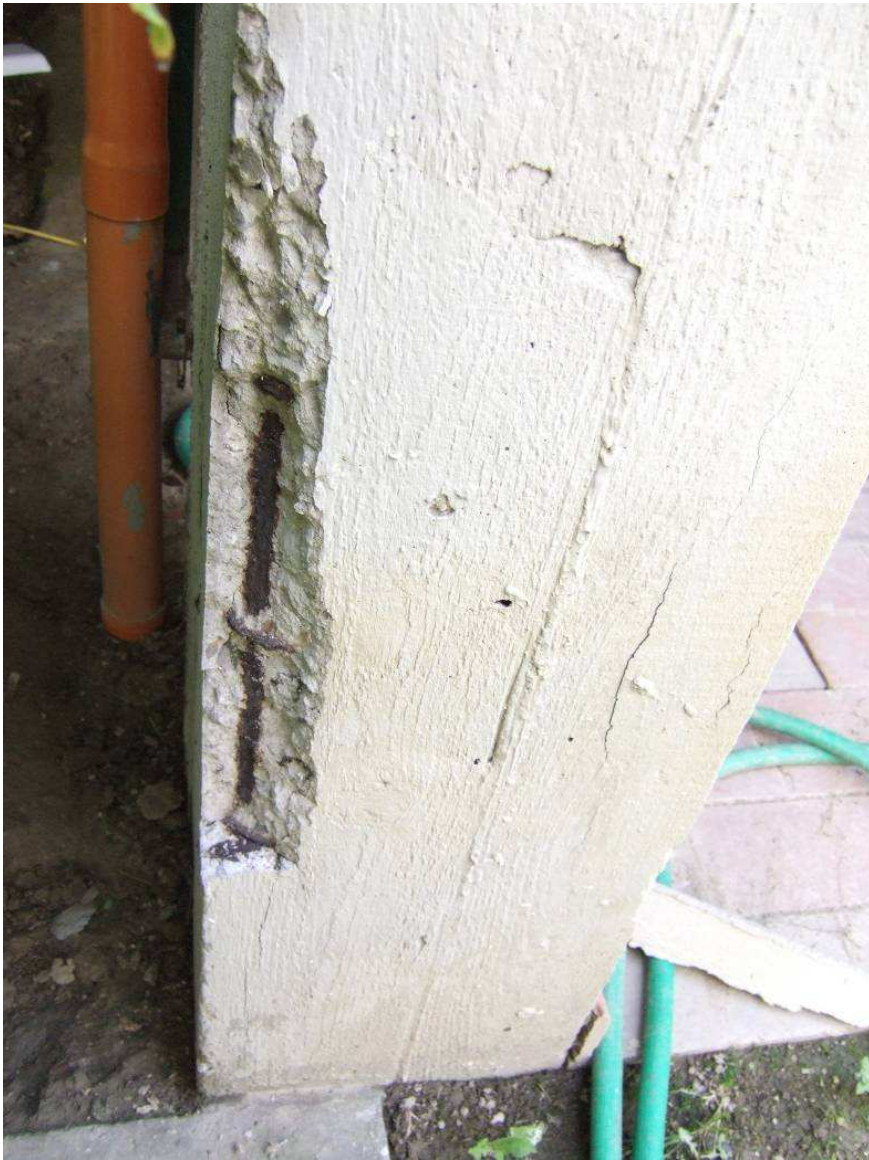
Corroded rebars
