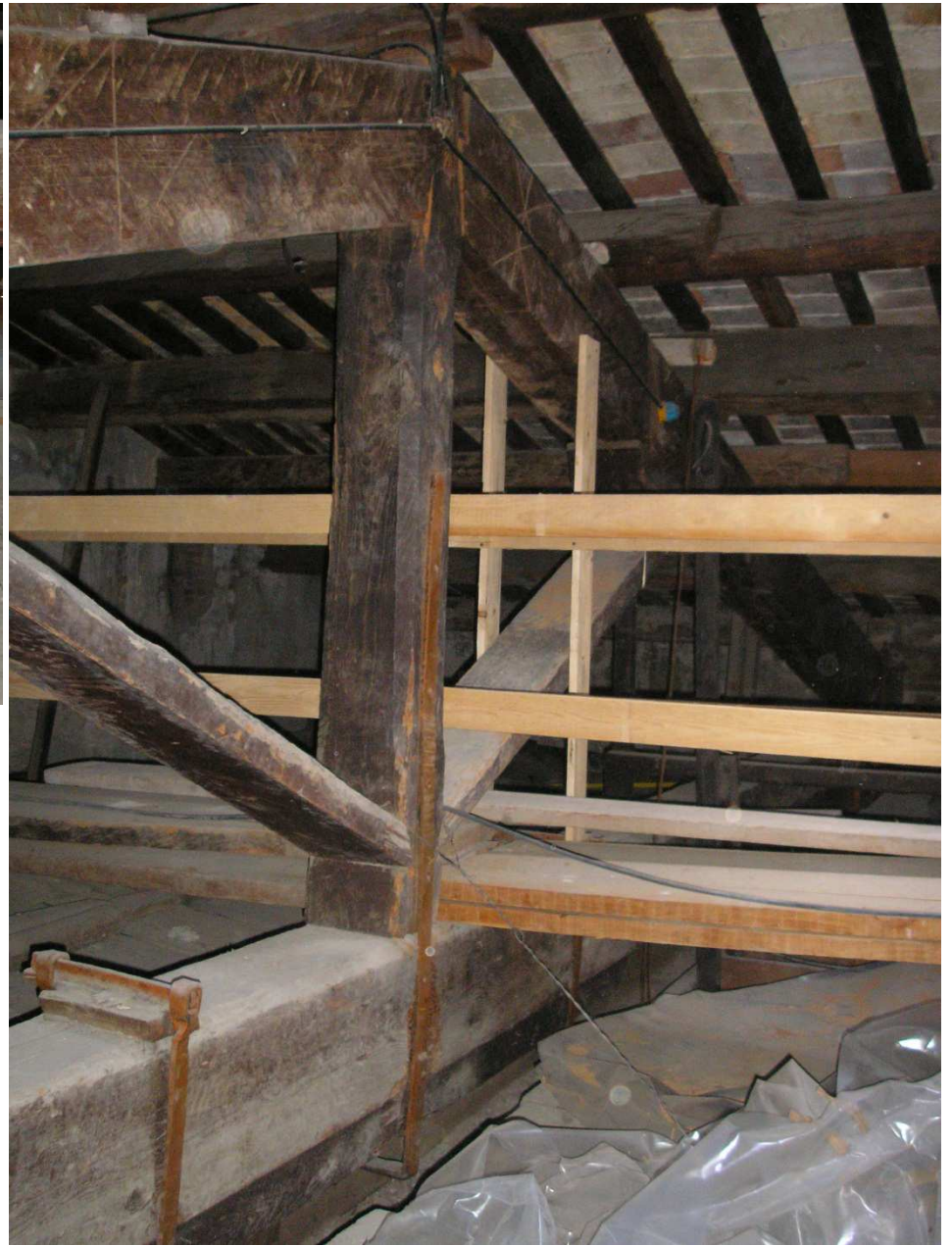
Suspension of the cieling
