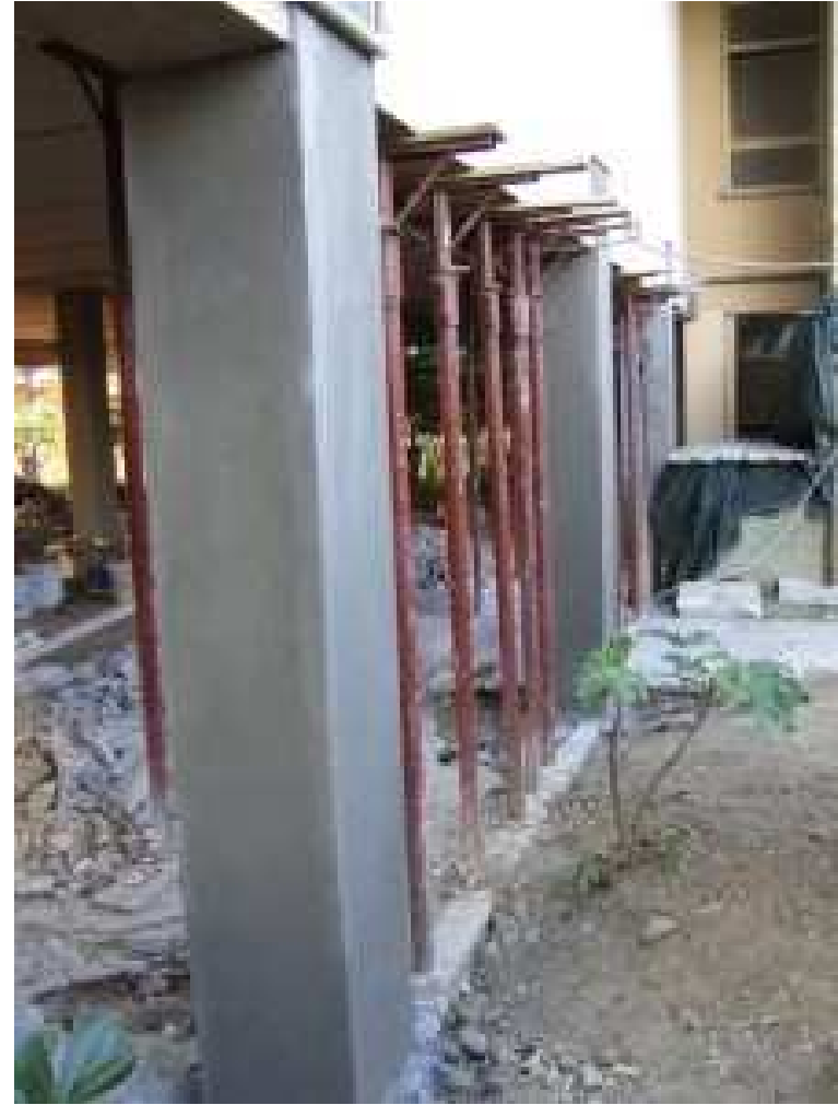
execution of the surface finish
