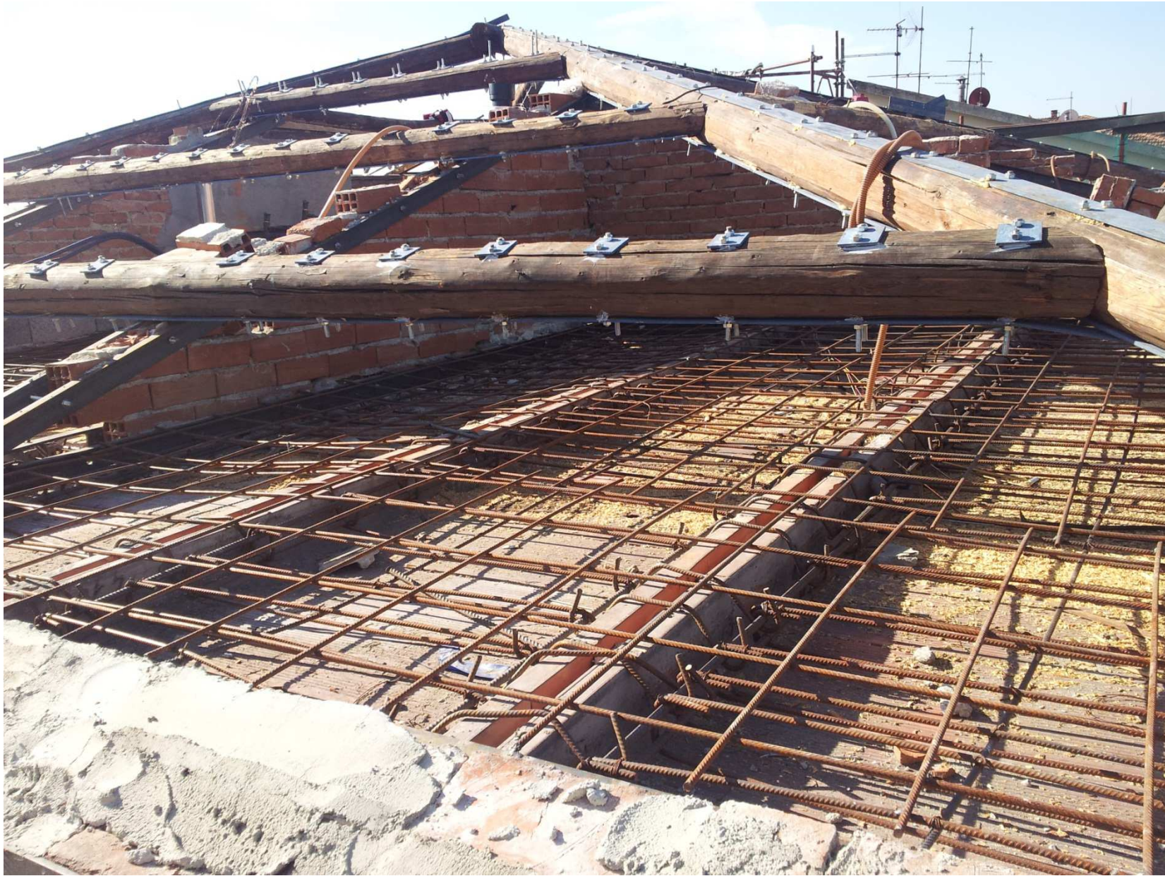
Strengthening of the roof during the works
