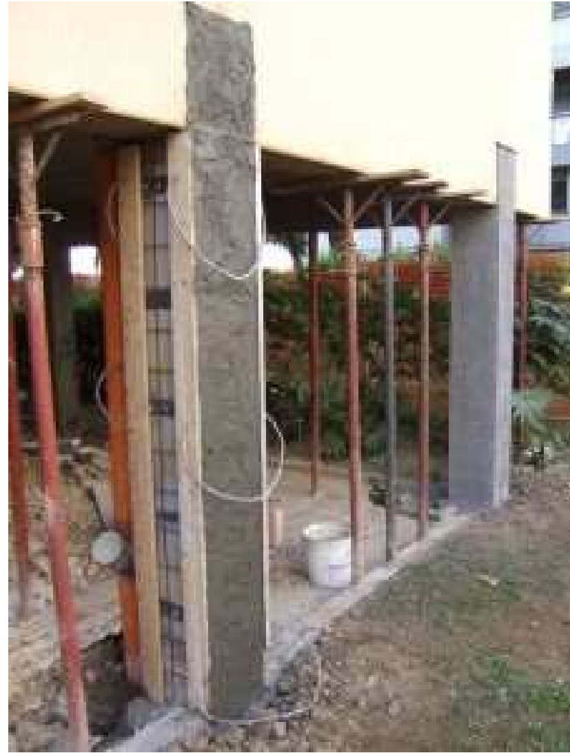
execution of the additional epoxy mortar layer ( s=50 mm)
