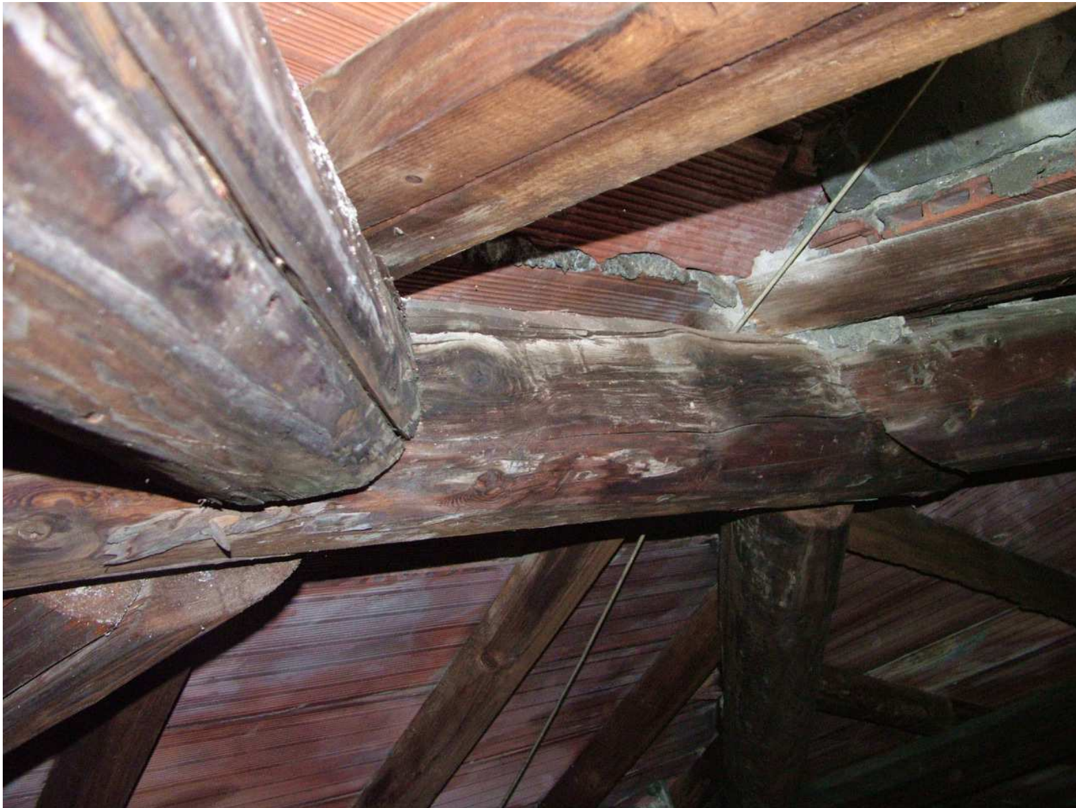
Connection between ridge beam and hip beams
