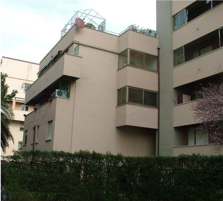
General view of the building
