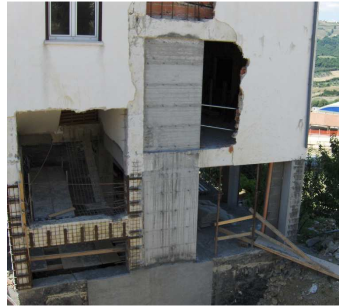
Execution of the shear walls
