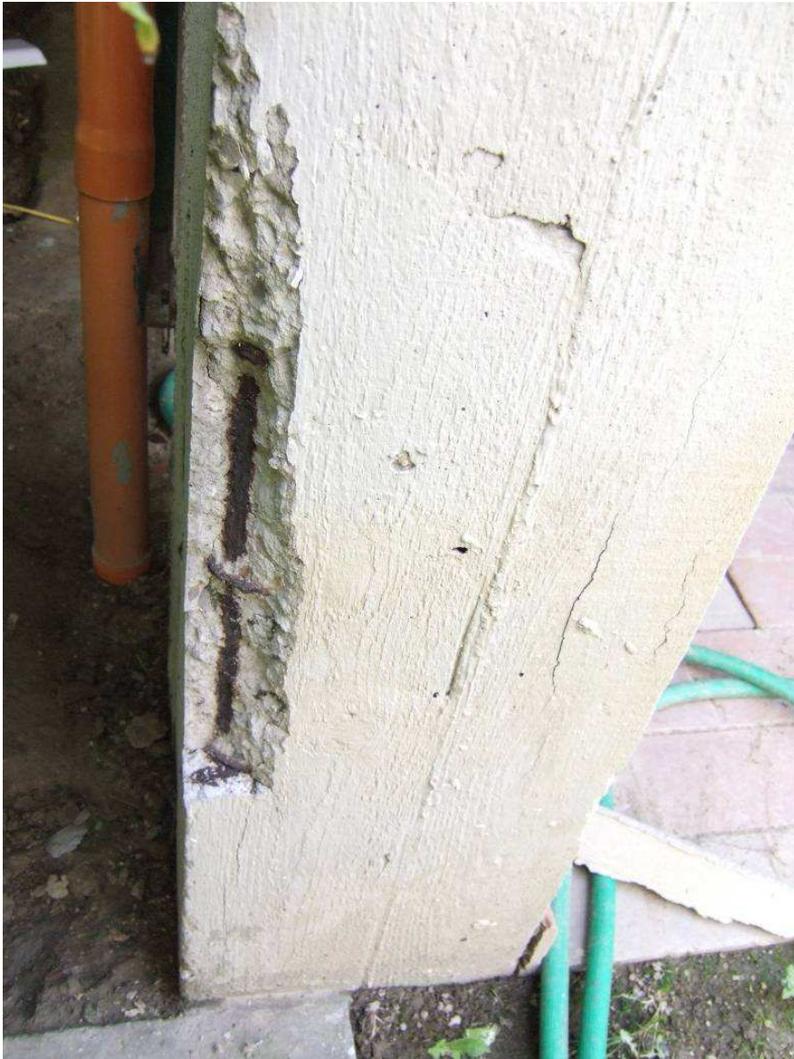
Corroded rebars
