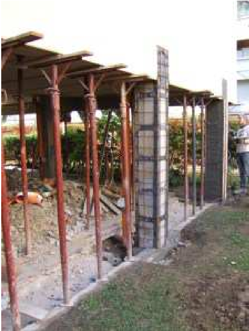
welding of steel mesh to the steel
