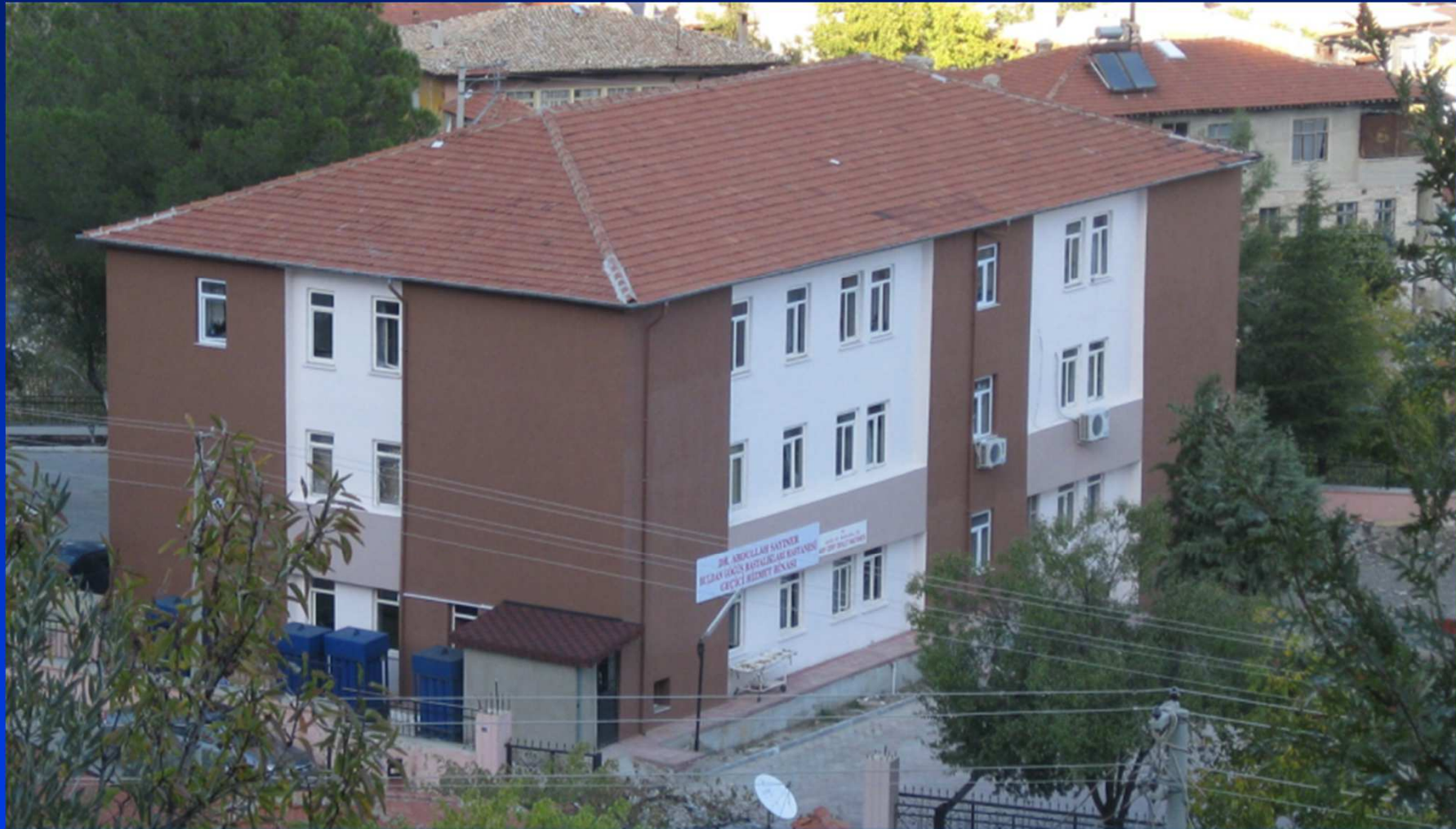
Same building after strengthening
